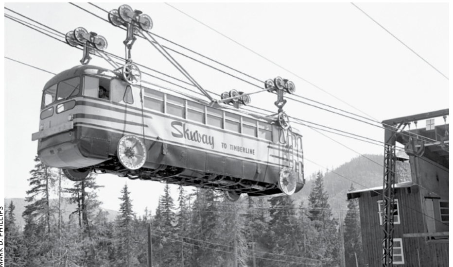
MARK D. PHILLIPS The Mount Hood Skiway launched in 1951. The enormous weight of the buses meant the lift hauled 72 skiers per hour—when a chairlift of that era transported 1,000 skiers in the same amount of time. The Skiway—which “proved to be not the most successful lift, but it certainly looked cool” as noted by a lift blogger—closed in 1956.
