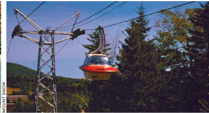
Installed in 1964, Mount Snow's Air Car delivered skiers in futuristic style for about 12 years.
