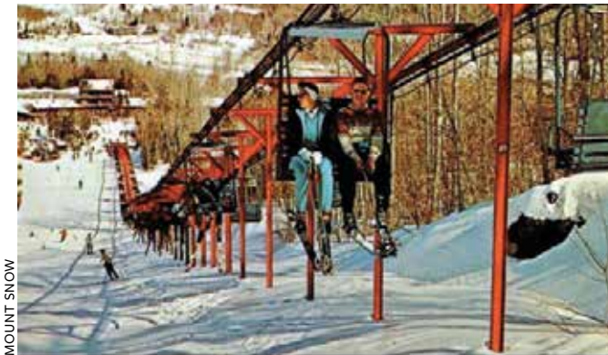
Called the "Clickety-Clack," the chain-driven Mount Snow lift didn't win any fans as it chronically dripped grease onto riders.
