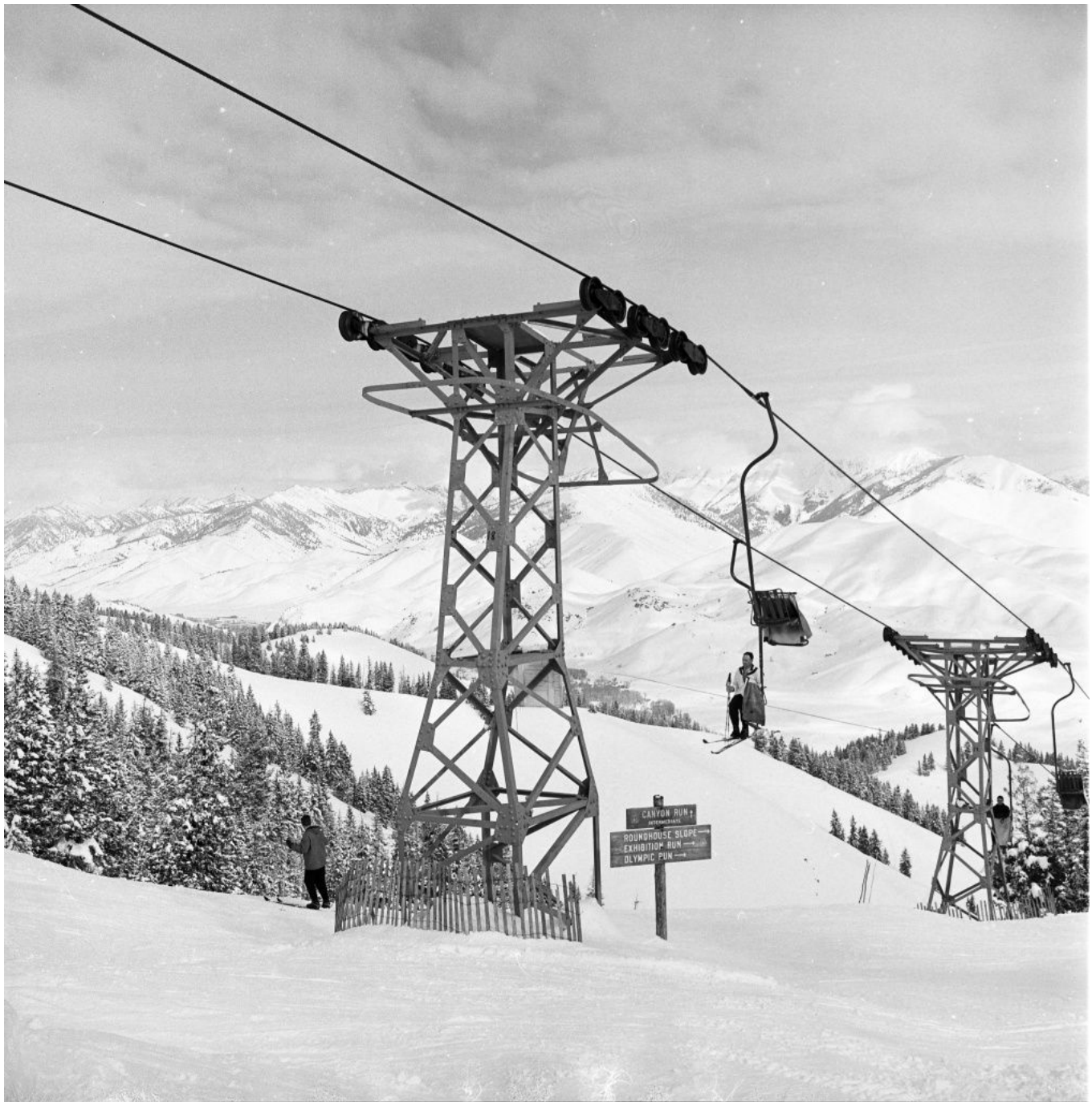
On the much taller Bald Mountain, they built three additional single-chair lifts that could help skiers climb nearly 3,400 vertical feet. The second-generation ski lifts featured steel towers. (Sun Valley Resort)
