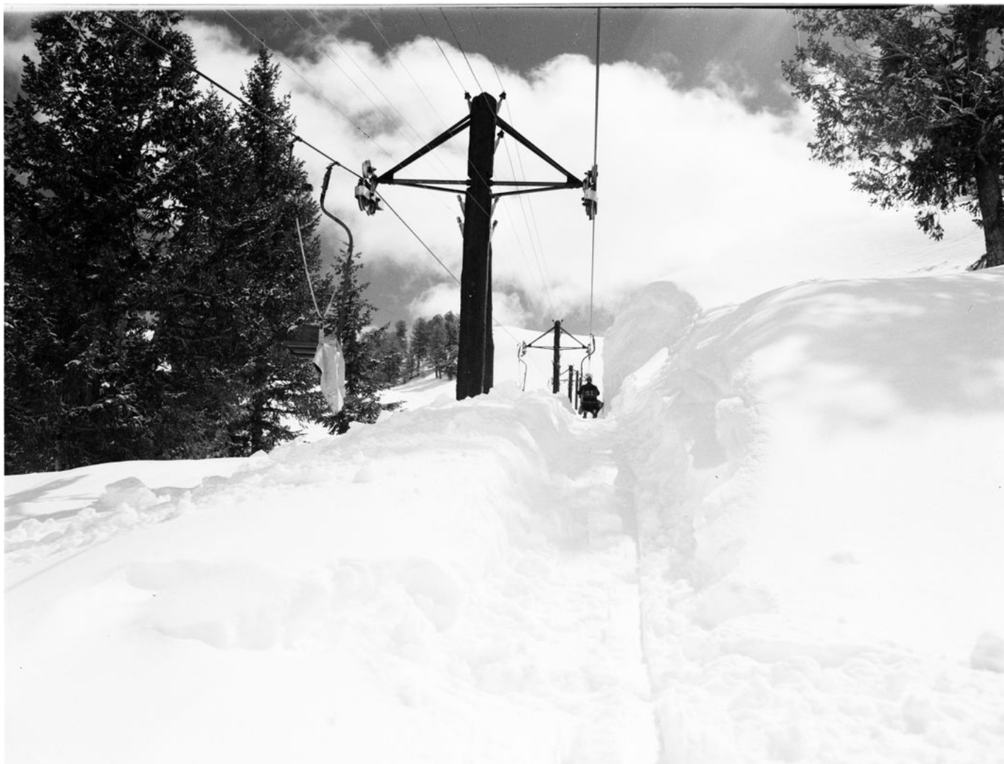
The original Proctor lift transported skiers, seated in chairs suspended 20 feet off the ground, for 3,540 feet and gained 1,150 feet in elevation. (Sun Valley Resort)
