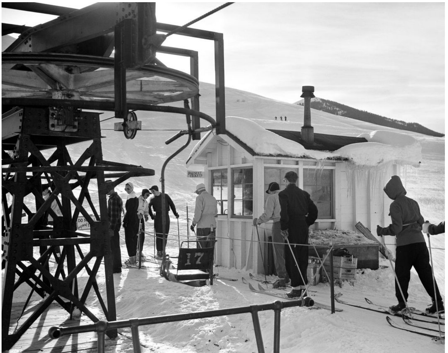
The Dollar lift was 2,360 feet long and rose 634 feet in elevation. (Sun Valley Resort)
